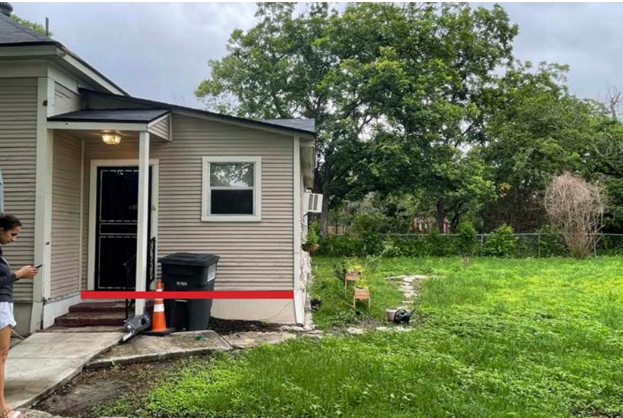
Addition to home to be removed. The roof will remain and this portion will become a back porch. These are all non-historic aluminum windows. The ogee siding which remains in good condition may be reused for repair and infill at other locations in the home.
