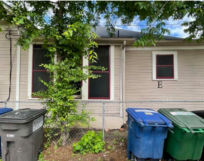
Window E to be removed and replaced by historic window located on the interior of the house labeled window 2 on schedule and demo plans.
