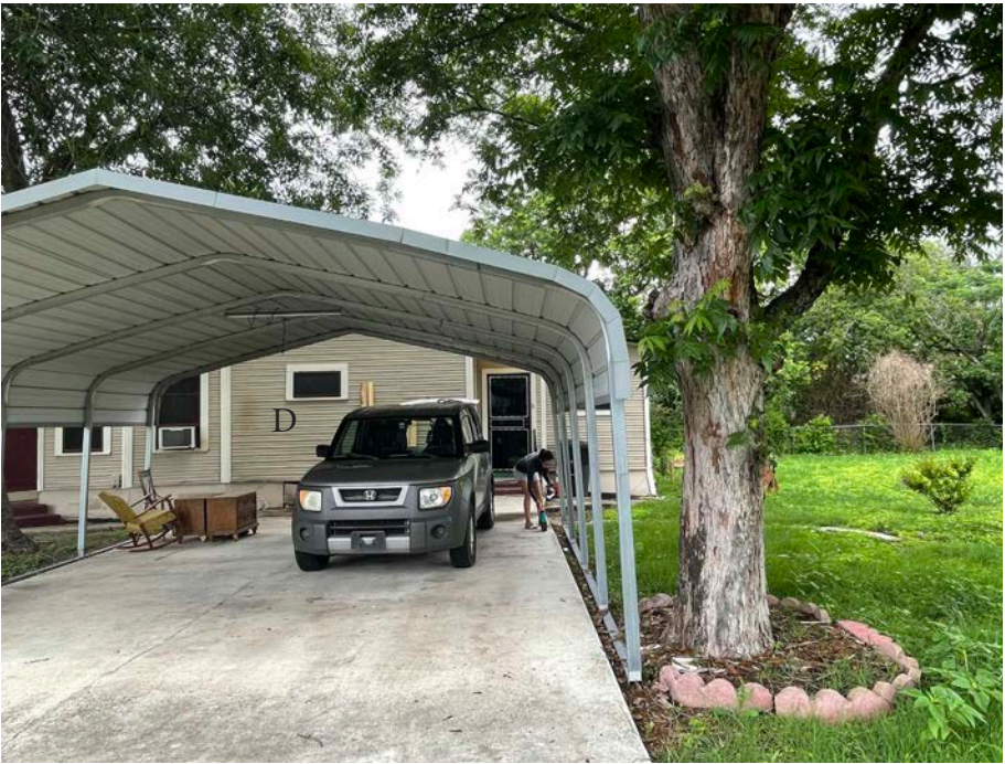
Window D to be removed and replaced with custom wood window to match existing windows. Labeled 3 on the plan and window schedule. Remove existing carport.
