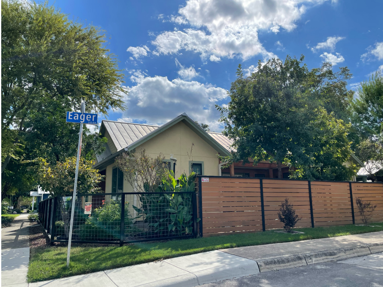
Example of 4' high Metal post and mesh gate and 6' high metal post and wood fence.
