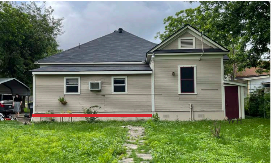
Addition to home to be removed. The roof will remain and this portion will become a back porch. These are all non-historic aluminum windows. The ogee siding which remains in good condition may be reused for repair and infill at other locations in the home. Water Heater Shed (WH) to be removed.
