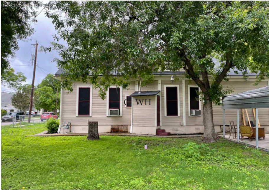
The water heater shed (WH) is to be removed and a new bay window will be placed back to it's original location. This window will be a custom wood window to match the other bay windows. Labeled window 1 on window schedule and floor plans. Window C will be removed and replaced by door for side yard access. Labeled Door 1 on floor plans and door schedule.
