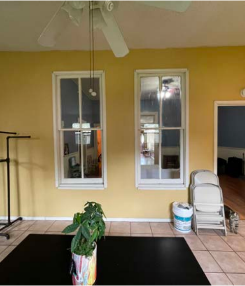
Exterior view. Window at interior location to be removed, and reused at exterior locations. Labeled window 2 on floor plans, demo plans, and window schedule.
